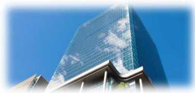
Grand Front Osaka Tower B 27th Floor
