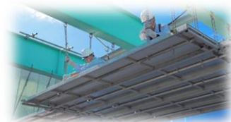
Panel hanging scaffolding SPIDER PANEL
