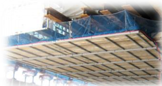
System hanging scaffolding VMAX
